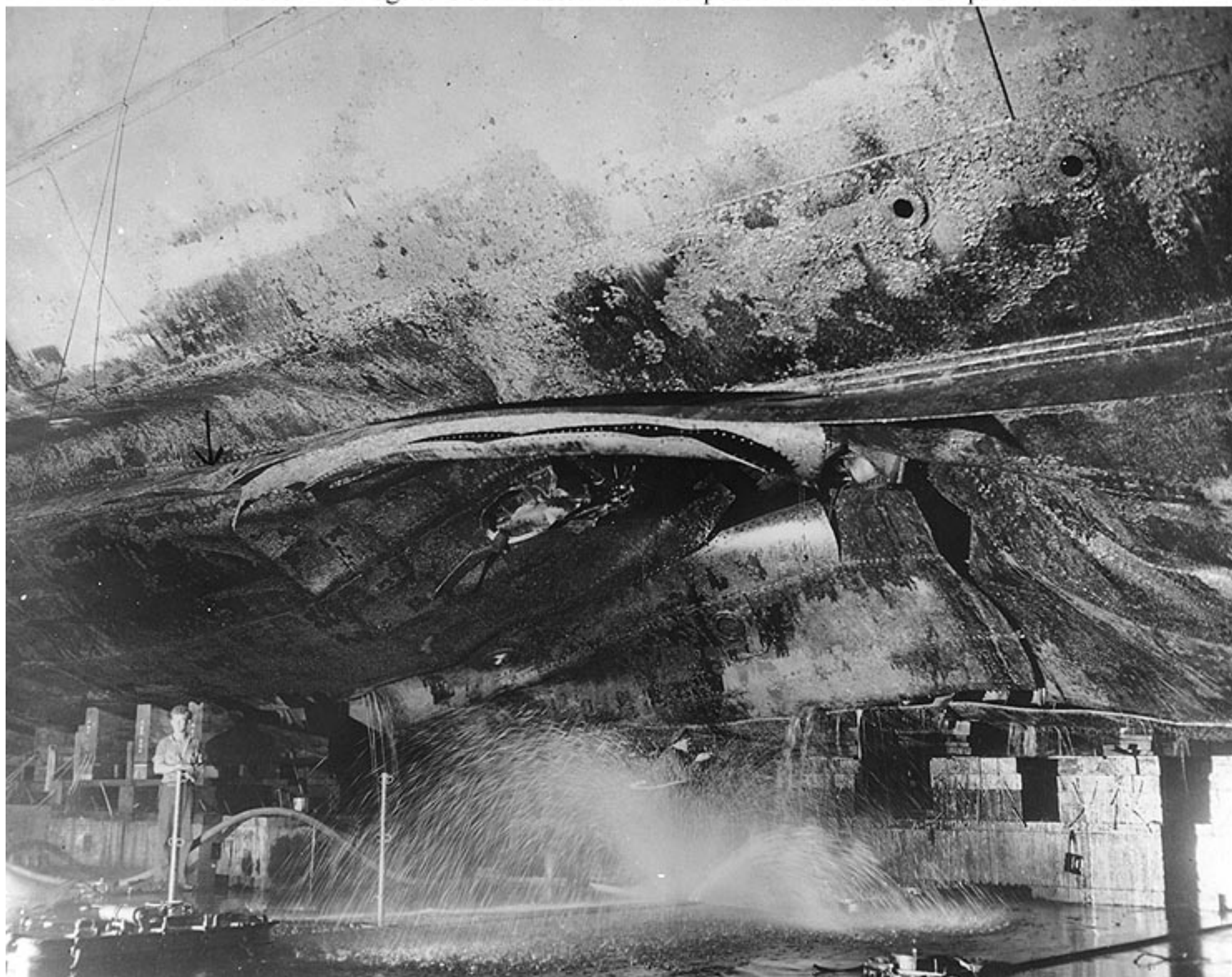
Photo # 19-N-105803 Damage to USS Houston from a torpedo that hit her amidships on 14 Oct. 1944
