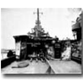
Photo 53: NEWCOMB (DD 586) Looking at forward end of replacement main deck plating.
