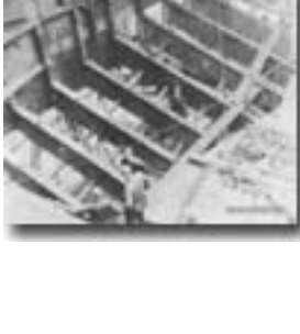
Photo 15: HOUSTON (CL 81) Repairs installed at Ulithi in way of after damage. Note shell plating and girders at main deck.
