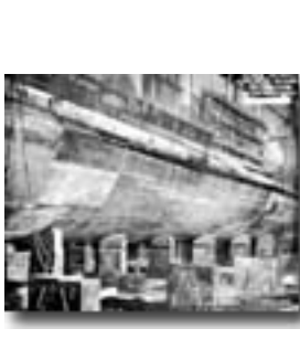
Photo 44: WADLEIGH (DD 689) Looking forward at replacement continuous longitudinals, intercostal transverse web frames and repaired bulkhead 110.
