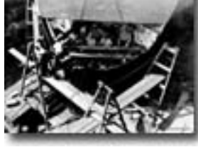
Photo 63: SELFRIDGE (DD 357) View while drydocked in ARD-2, after removal of below water structure and during process of installing stem and supporting girder.
