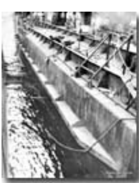
Photo 55: NEWCOMB (DD 586) Looking forward along port side at T stiffeners installed on shell and deck plating.
