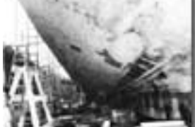
Photo 9: RENO (CL 96) Looking forward at after end of replacement plating. Note watertight seal on port stern tube.
