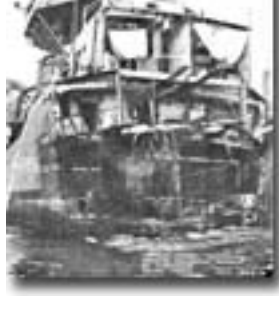
Photo 59: SELFRIDGE (DD 357) View of bow after removal of wreckage and start of temporary repairs.
