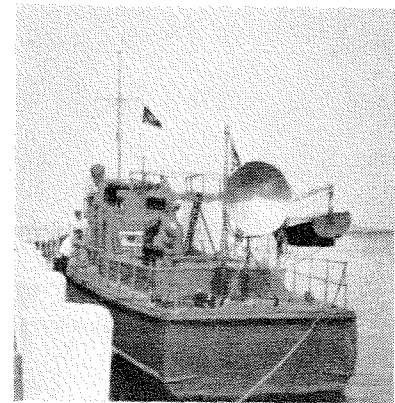
Fig. 5—Early experiments by Signal Corps Laboratories on 9-centimeter continuous-wave equipment located on Signal Corps boat. August, 1934.
