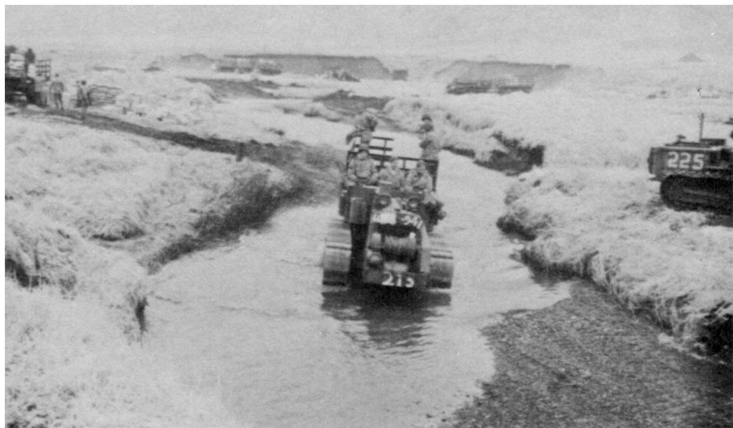
INGENIOUS USE OF TERRAIN FEATURES by individual units facilitated the delivery of supplies and equipment. The gravel bed of a stream used as a road when equipment bogged down in the tundra on Attu (above), and a roadside bank used as a loading ramp in Australia (below).
