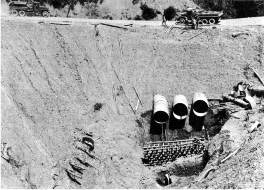
DRAINAGE CULVERTS are installed on the Ledo Road.
