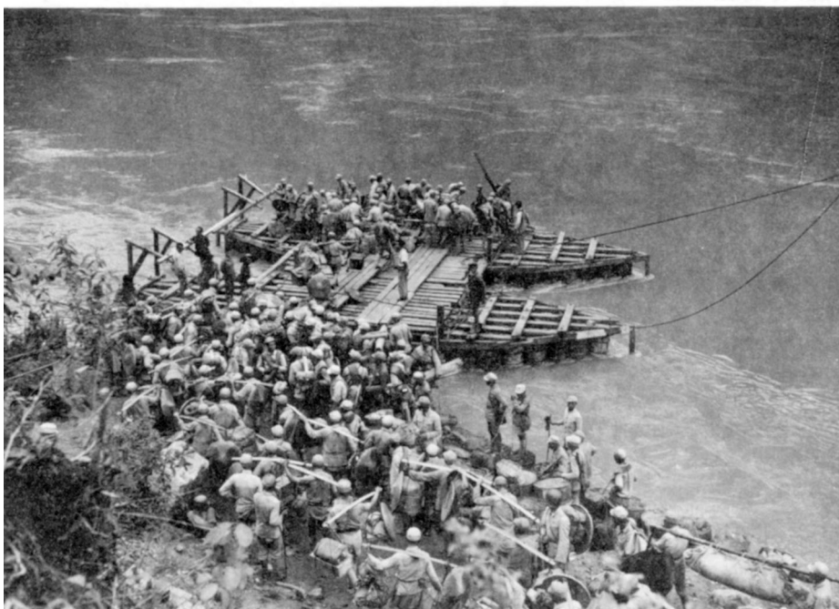
CHINESE TROOPS CROSS THE SALWEEN, in rubber boats (above), and by means of a ferry constructed from oil drums (below).
