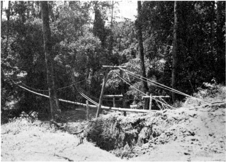
PIPELINE CROSSING A STREAM by means of cable suspension.
