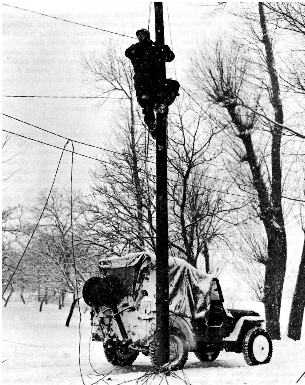
SIGNAL LINEMEN REPAIR WIRE IN THE ARDENNES
