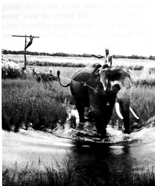
ELEPHANT DRAWS WIRE TAUT during pole line construction near Shampur, India. 31st Signal Construction Battalion.
