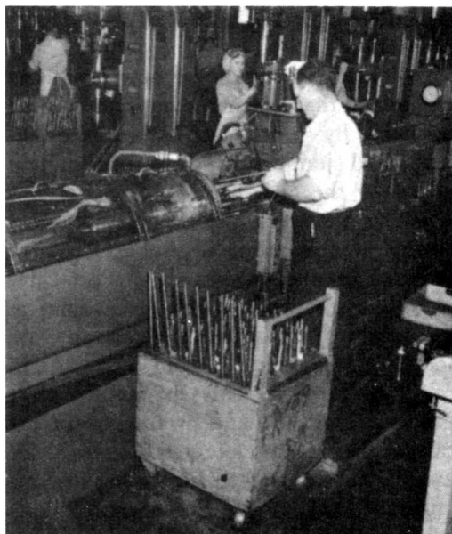
PRODUCING CARBINE BARRELS. Finished barrels ready for the assembly department (left); broaching the rifling grooves in the carbine barrels (right).
