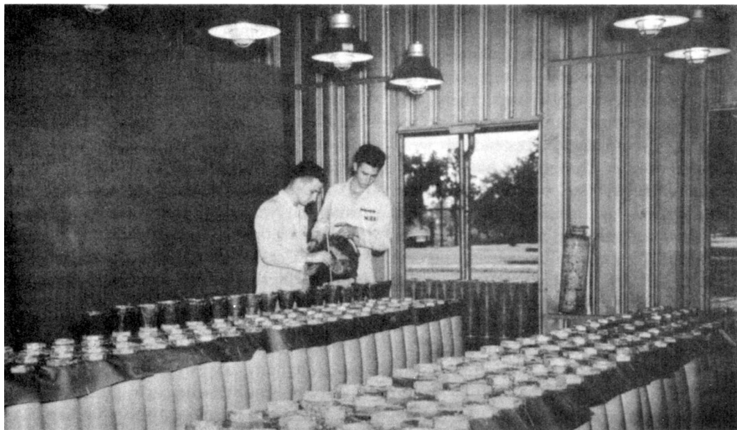
WORKMEN POURING MOLTEN TNT INTO 155-MM. SHELLS at Charleston Ordnance Depot, October 1941.
