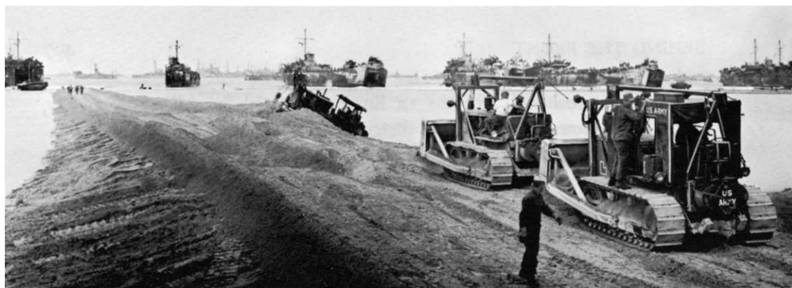
Ship-to-shore supply causeway at Hagushi beaches
