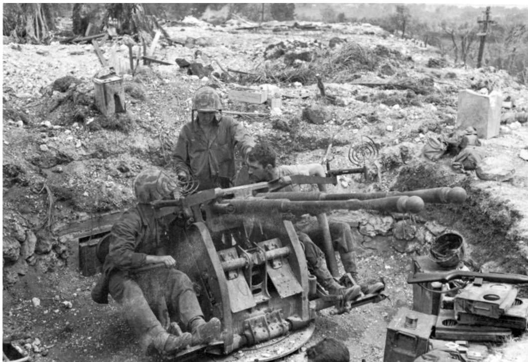
JAPANESE TYPE 96 25-MM. MACHINE CANNON. U.S. marines repaired this damaged twin-mount weapon fitted with speed ring sights and promptly put it to use against the enemy.
