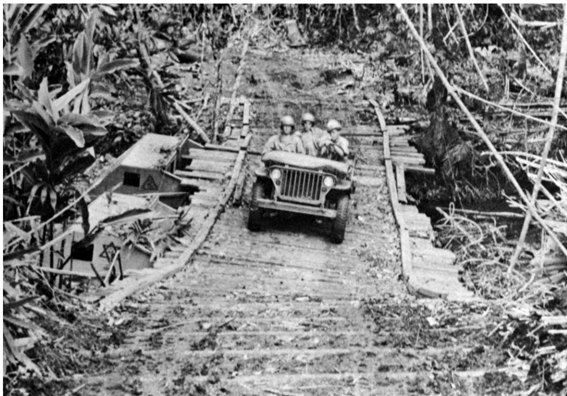
BRIDGING THE TENARU RIVER, amphibian tractors were used to support the flooring as the Marines moved to expand the beachhead 7 August.
