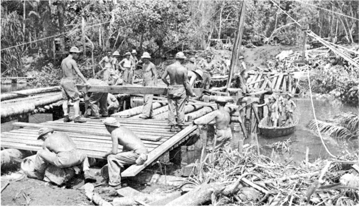
BRIDGES AND ROADS in Guadalcanal were virtually non-existent when American forces landed. Engineers used native materials, supplemented by imported materials (above) to put a permanent bridge over the Matanikau River, but were unable to do much about jungle roads (below) when it rained.
