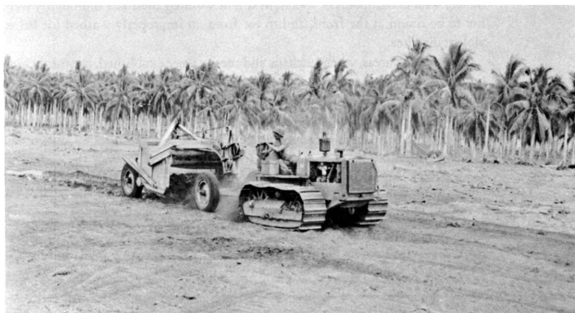
CONSTRUCTION EQUIPMENT was scarce and inadequate. The light bulldozer above is shown improving the trail over "Windmill Hill" (Hill 35) on Wright Road. Runways were leveled by small Army Corps of Engineers earth movers which had been brought to Guadalcanal only when already-crowded transport space would permit.
