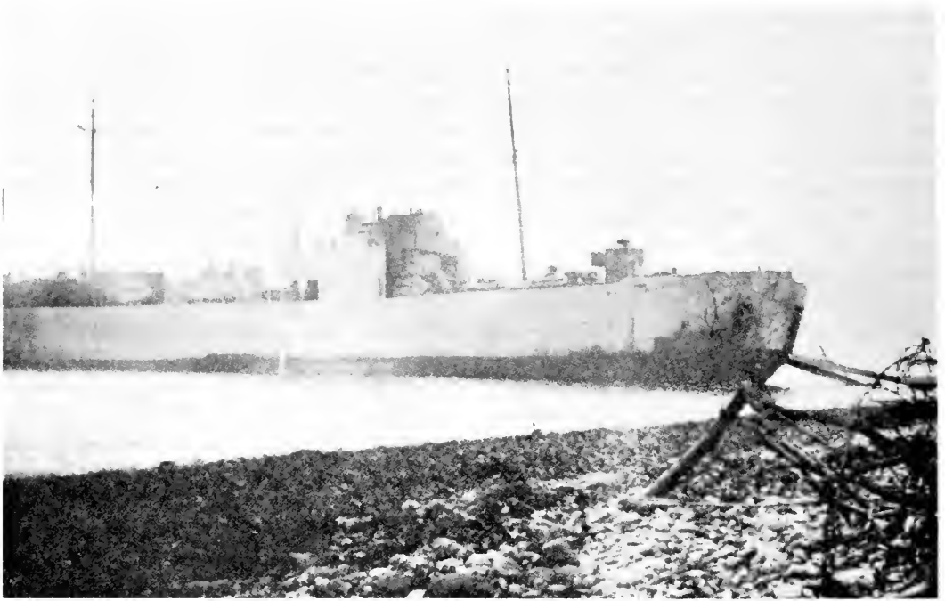
THE “MARACAIBO” H.M.S. MISOA, October 1942. This was one of the three converted shallow-draft oilers used as tank landing ships at Oran. Note bridge sections from ship to shore.
