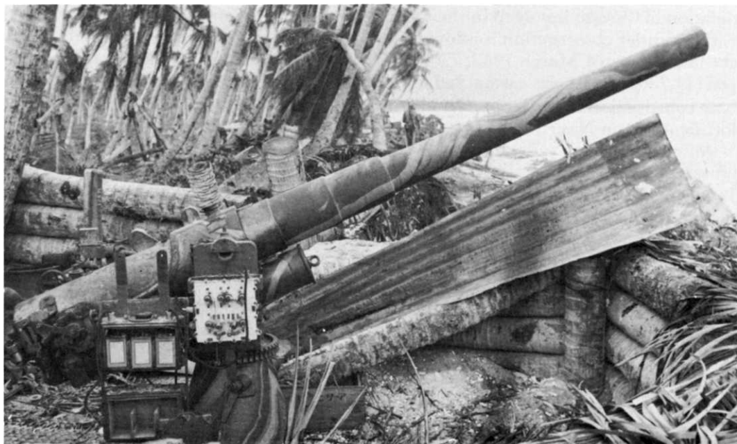
JAPANESE COASTAL DEFENSES. 8-cm. naval guns installed in log emplacements on Makin (above) and Tarawa (below).
