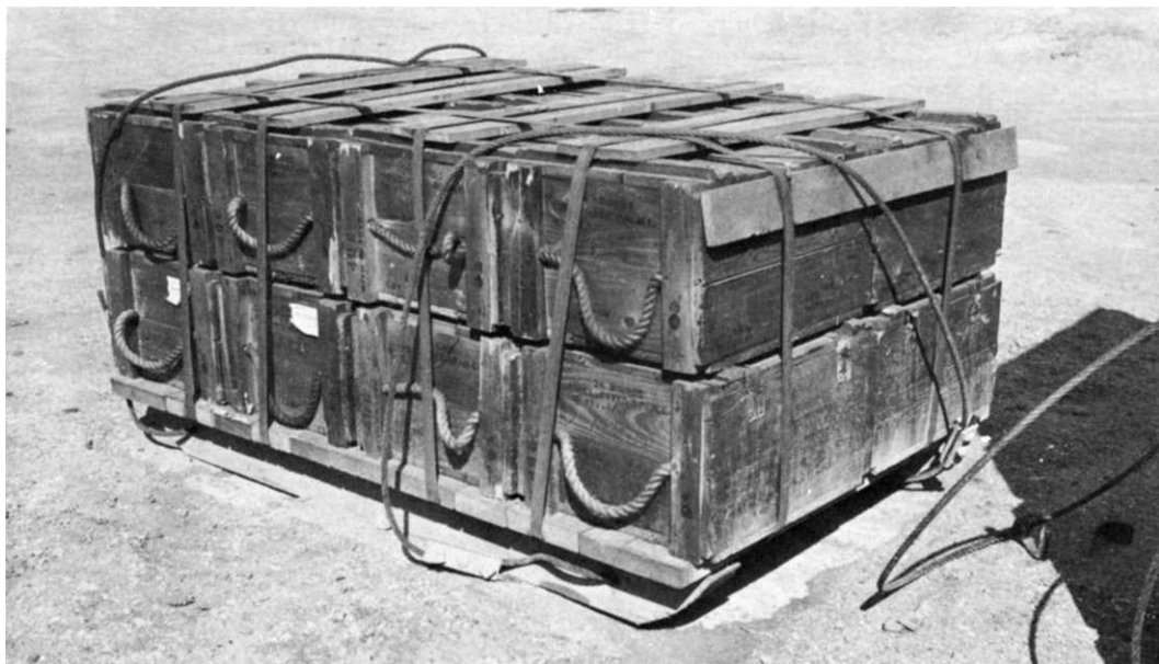
SUPPLIES PALLETIZED for the Gilberts operation . Method of loading and strapping (above); an LVT towing a loaded pallet during the actual operation (below).
