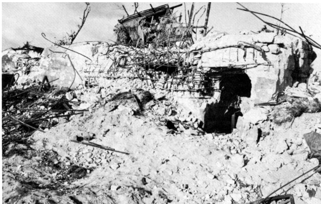
JAPANESE BOMBPROOF SHELTER of reinforced concrete and steel. Note steel door visible in the lower part of the entrance.
