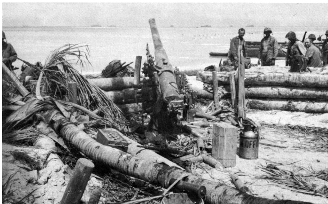
JAPANESE COASTAL DEFENSES. 8-cm. naval guns installed in log emplacements on Makin (above) and Tarawa (below).
