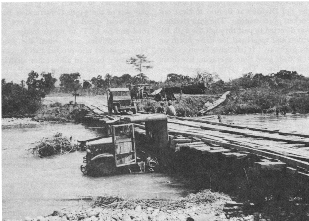
ENGINEERS USE A JAPANESE TRUCK TO SUPPORT A TEMPORARY BRIDGE in the Cagayan Valley.
