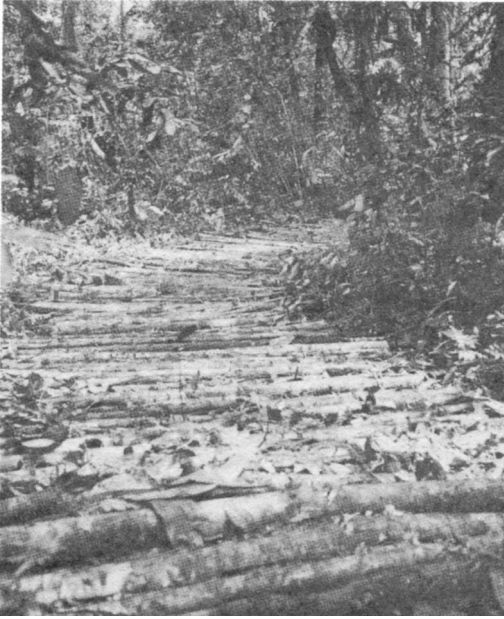
A CORDUROY ROAD, NEW GEORGIA, capable of supporting 155-mm. howitzers.
