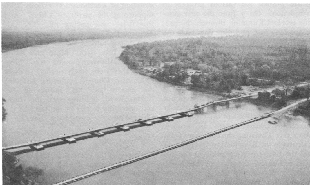
THREE EXAMPLES OF BRIDGING IN THE CBI. Above, the steel barge bridge across the Irrawaddy, with a temporary ponton bridge in the foreground. Below, the Bailey suspension over the Taping River.
