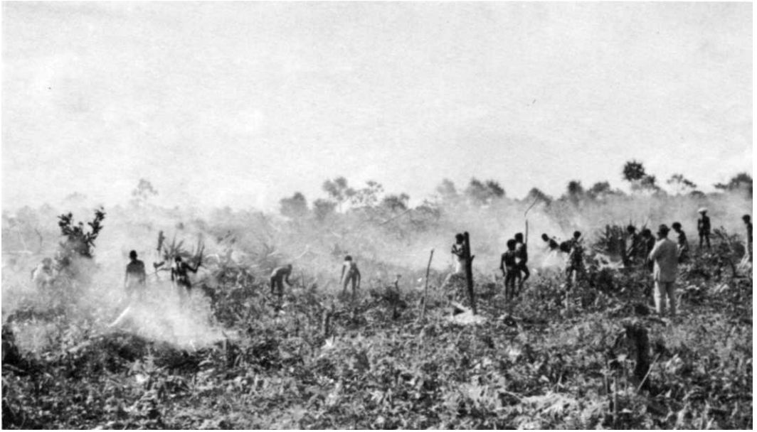
CLEARING AIRFIELD SITE WITH HAND TOOLS, Kiriwina Island, July 1943.
