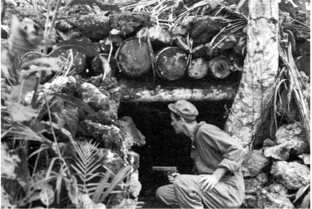
PILLBOX MADE OF COCONUT LOGS AND CORAL near Munda Airfield.
