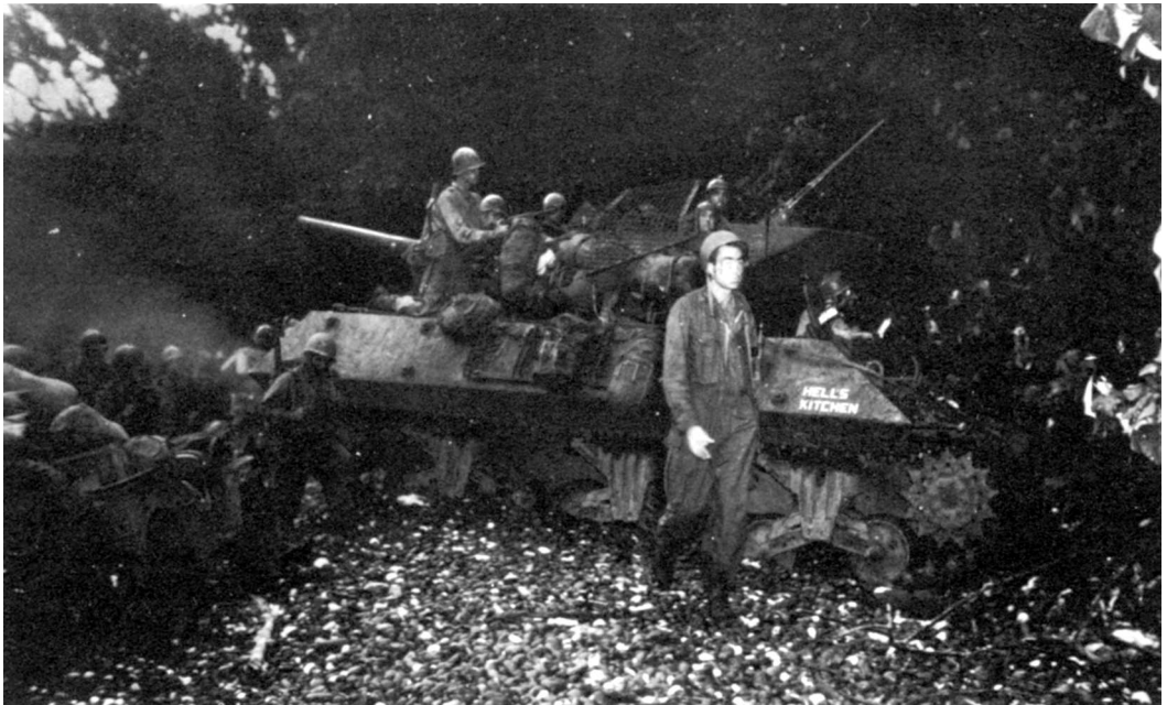
M10 MOTOR CARRIAGE MOUNTING 3-INCH GUN on a rough and stony beach near Saidor, 2 January 1944.
