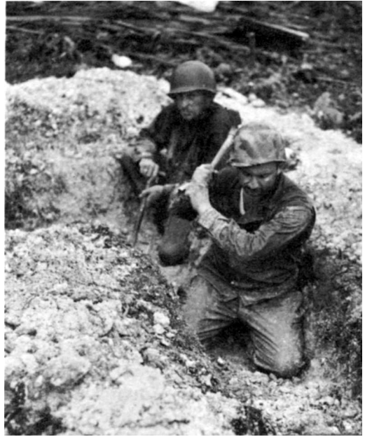
DIGGING A FOXHOLE THROUGH CORAL ROCK near the airstrip, 29 February 1944.
