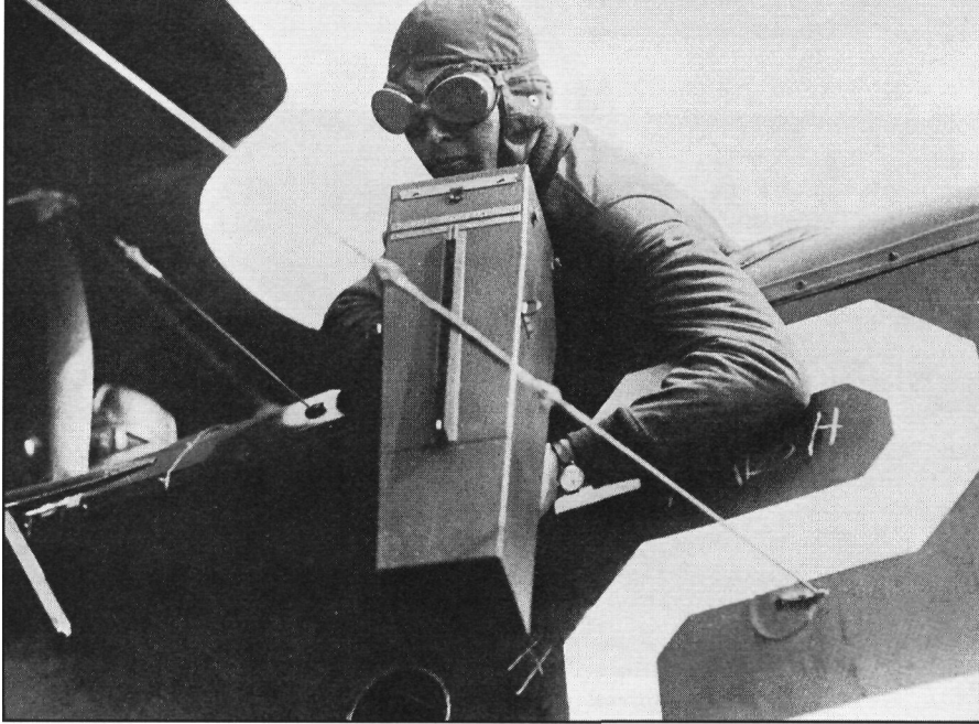
Aerial photography permitted precise targeting throughout the theatre and up-to-date mapping of ever-changing trenches. Here an observer operates the Graflex camera from an observation plane.
