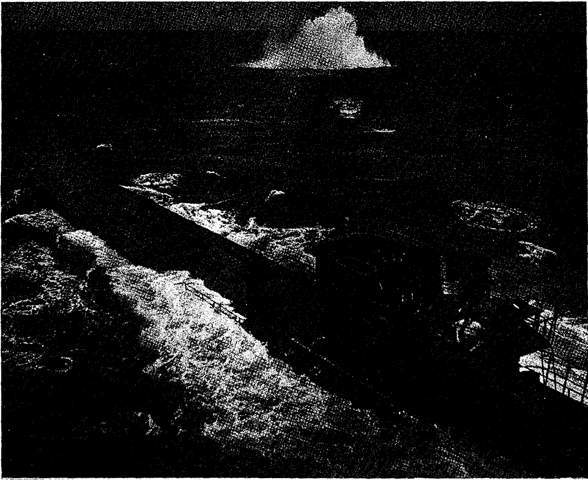
FIGURE 5. Attack by U. S. Navy Liberators (VPB-107) between the coast of Brazil and Ascension Island, November 5, 1943. Note the radar antenna in its fairing on the left side of the conning tower, and just forward of it, an early form of the Naxos search-receiver antenna. The guns are still pointing at the previous position of the aircraft, while the gun crews seek cover from the 20-mm fire from the aircraft's turrets.
